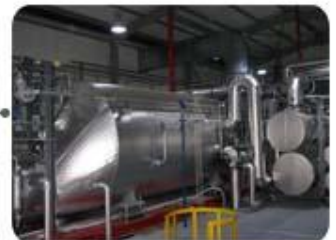
Chemical storage tanks
