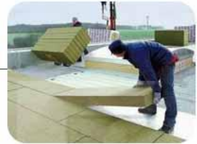
Roof Insulation
