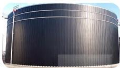
Tank Insulation Jacketing
