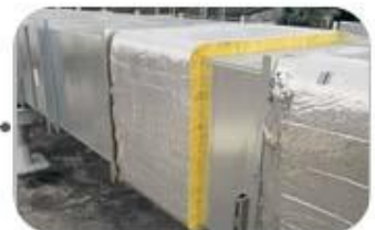
Industrial Tank Insulation
