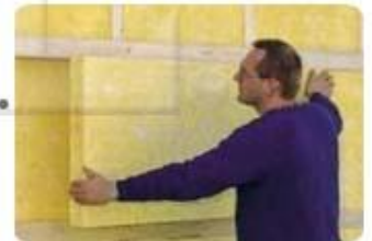
Cavity Wall Insulation
